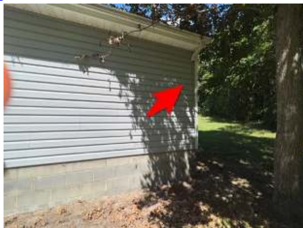
32: Missing downspout at the back right corner of the detached garage. Also, the gutter is pulling away from the fascia at the right front corner of the garage.- $200
