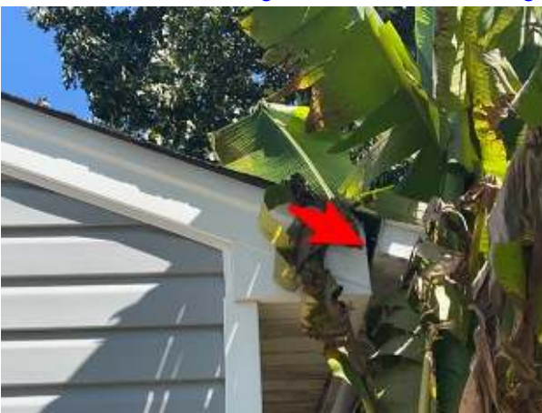
32: Missing downspout at the back right corner of the detached garage. Also, the gutter is pulling away from the fascia at the right front corner of the garage.- $200
