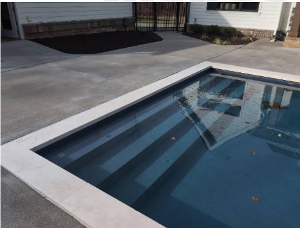
Missing handrail
